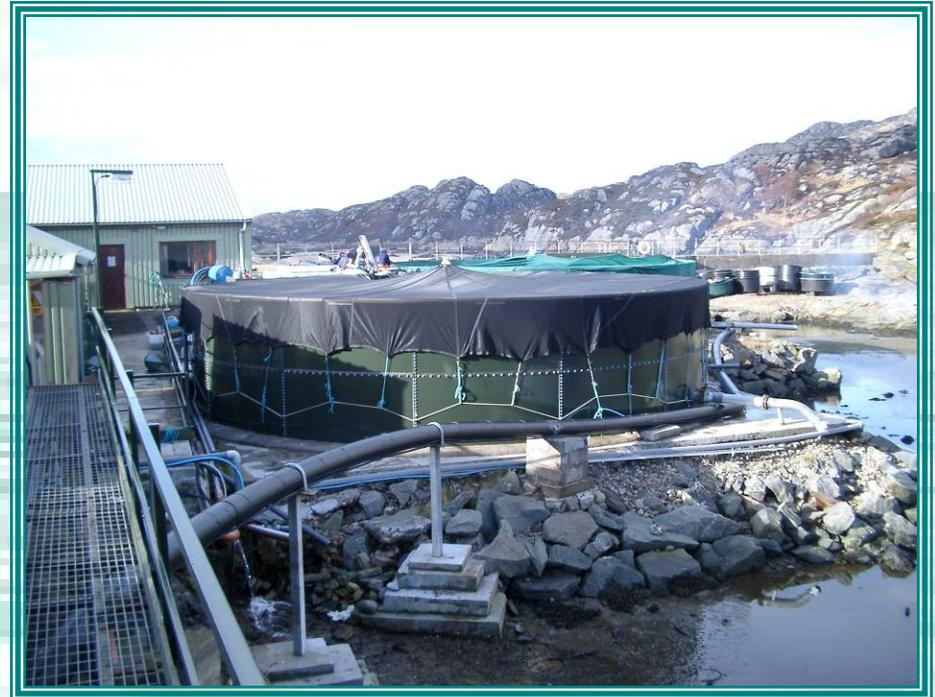
A 10 m diameter circular tank broodstock, with its own light-proof cover
