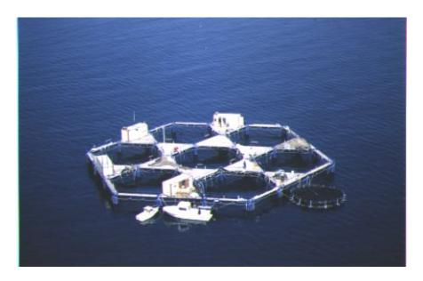
**Figure 37** Fish farm platform from Marina System Iberica – Cripesa. The basic structure is the same as the Pisbarca but incorporates an automated feeding system (http://www.msicom.net)
