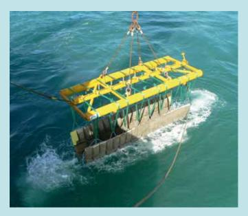
Concrete mattresses come in various forms, offering different degrees of flexibility and density to cater for different conditions and uses. But typical dimensions and weight are:
