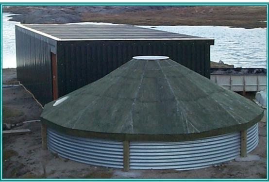
An example of a simple individually insulated fish tank, with a water recirculation system within a shed in the background - note the shed would be capable of housing treatment units for several tanks
