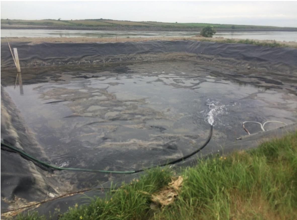
**Figure 6.** A 25 x 25 x 1.5 m spating pond at Carltron Point Hatchery in Ireland. Note the water outlet in far left-hand corner, this arrangement maintains water levels when flow is open.
