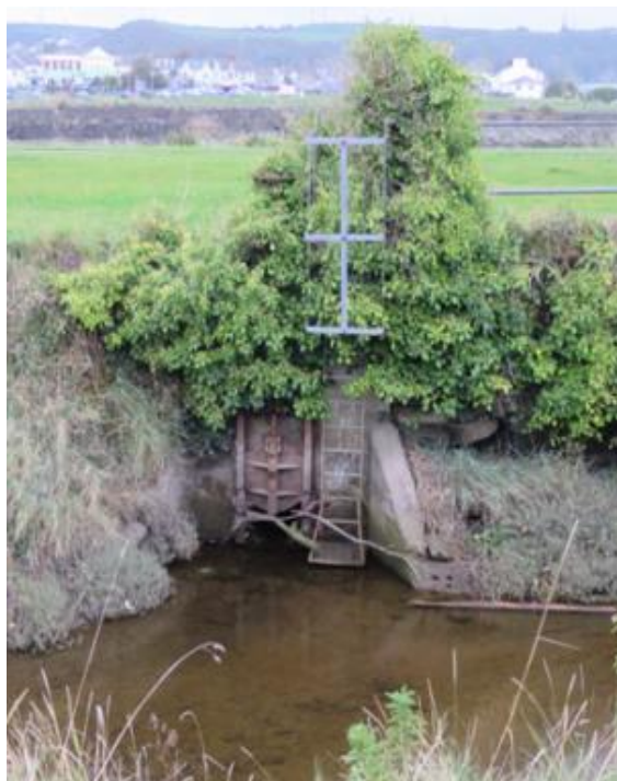
Plate 25: Combined sewage outfall (CSO) at Burry Port, Burry Inlet
