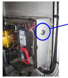
Temperature data logger fixed to switch box in engine room to capture ambient temperature (4). Loggers were set to capture the temperature at 60 minute intervals. Each logger holds approximately 5 months worth of data.
