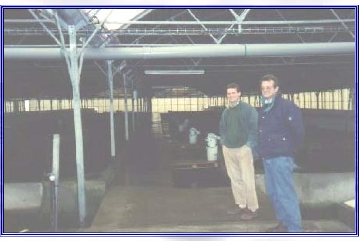
Cheaper forms of covered ongrowing units can be achieved by using "greenhouse" technology, but with rigid and opaque paneling. This unit also utilises concrete as the main construction material.
