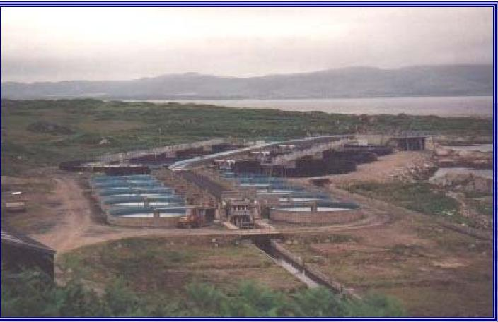
A typical marine fin fish land-based ongrowing unit. Located near the sea, with a large seawater pumping and screening system. Water is distributed to the tanks via a large open "flume" system, and effluent is discharged from the farm as far away from the seawater intakes as possible. Oxygen and aeration systems help to minimise the total pumping requirement.
