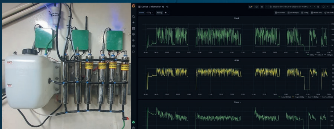
Left: An installed EcoPro system Right: Readings can be monitored live through the dashboard system
