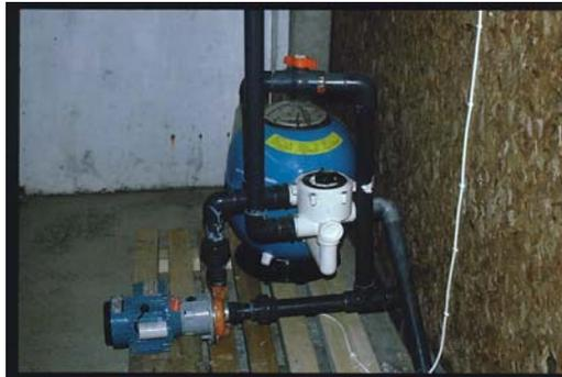
Plate 10: A sand filter used for mechanical filtration
