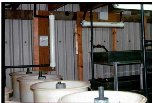
Plate 12: Individual wall-mounted UV units
