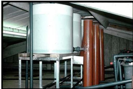
Plate 11: Simple biological filter towers and foam fractionators
