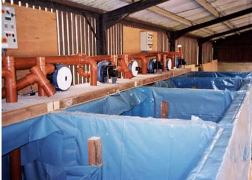
*Figure 10 – Photograph of woodchip and bark bio-filter facility during construction*
