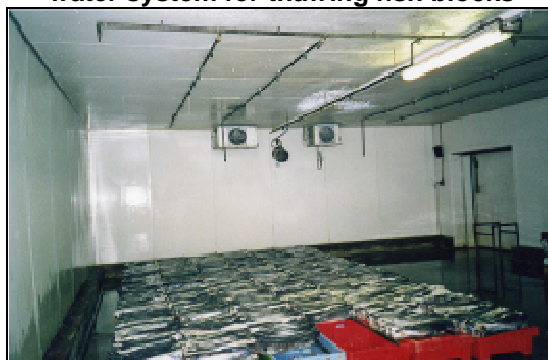
Figure 5 - An example of a simple spray water system for thawing fish blocks
