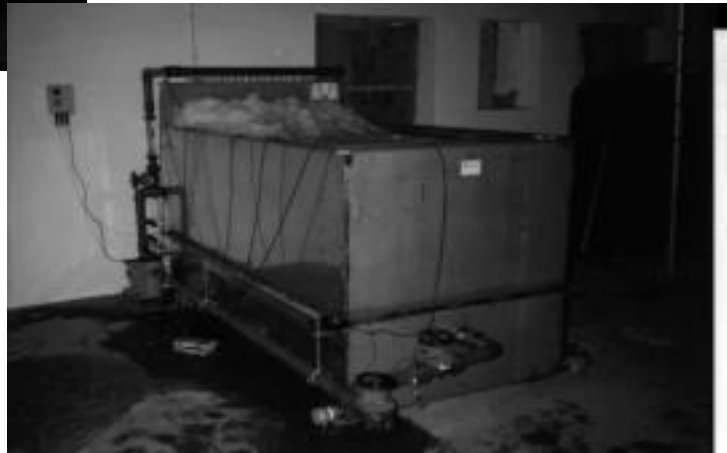
Stainless Steel Tank
