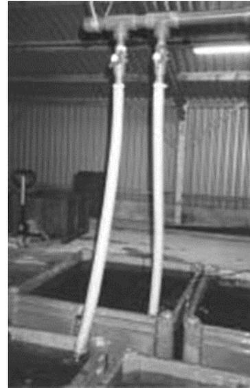
**Flexible feed pipes and control valves**
