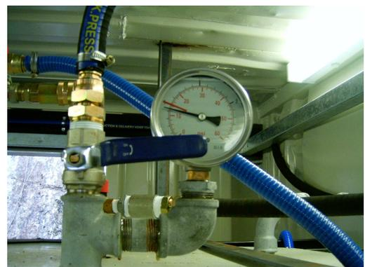
**Figure 11: The vent valve closed and the pressure nearing 1 bar.**
