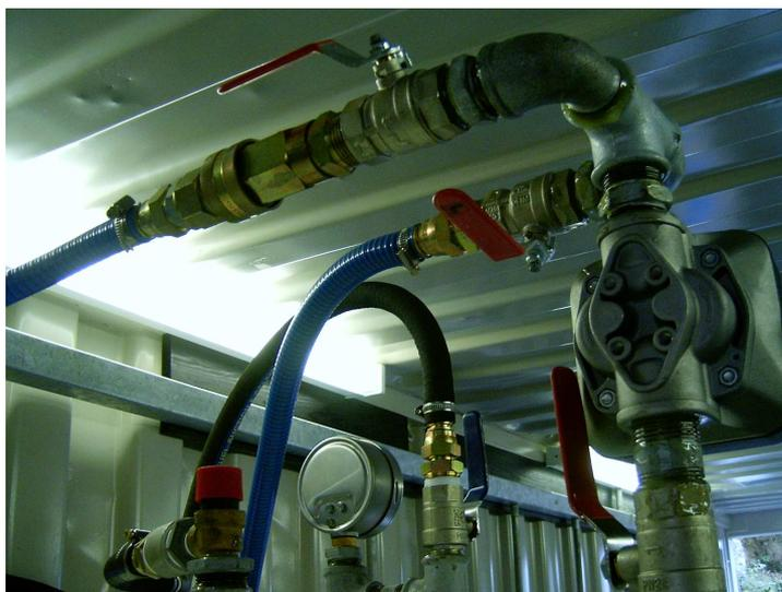
**Figure 9: Methanol delivery hose connected and 4 valves set for methanol delivery.**
