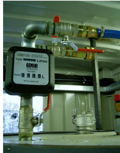
**Figure 10: The valves set for oil delivery.**
