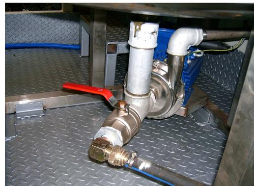
**Figure 13: The valve beneath the reactor closed**
