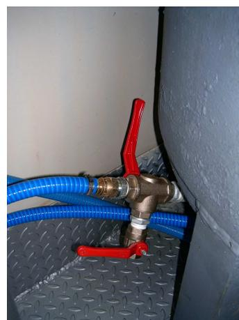
**Figure 15: The glycerine slug valve and the methyl ester outlet valve (both closed).**
