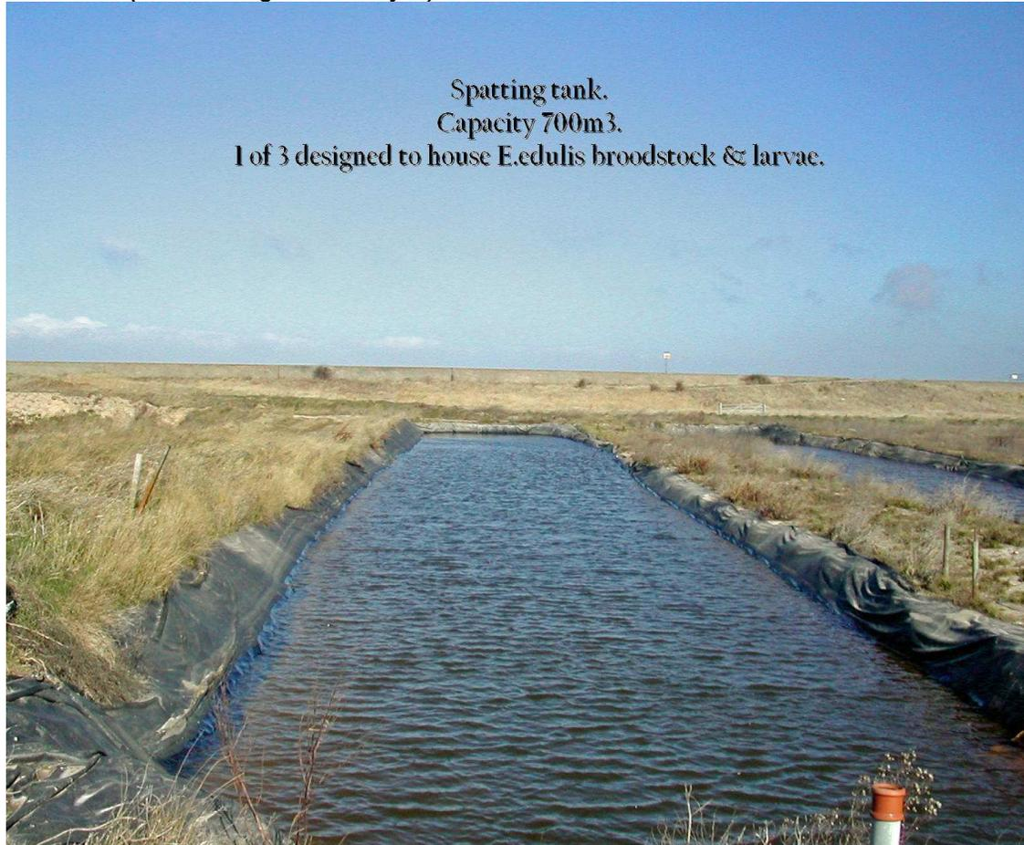
The pond image shown in Figure 17 shows how the butyl rubber liners have continued to remain functional and watertight after three seasons.
