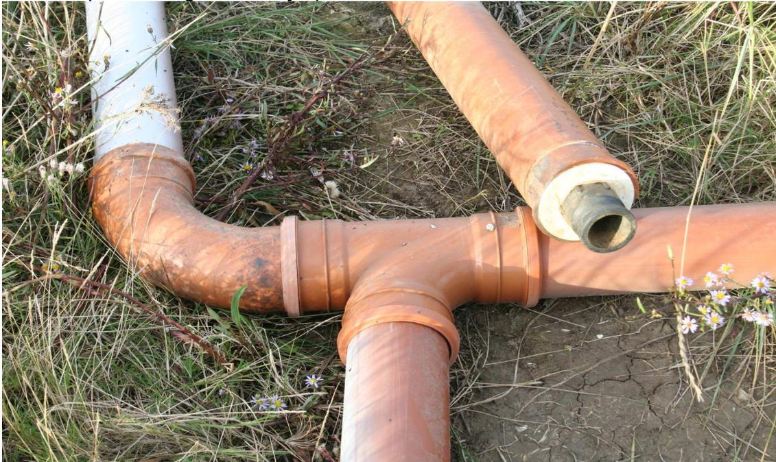
These 110mm pipes are less expensive than the 62mm polythene pipe and are readily available from any hardware supplier. These pipes are not liable to bursting as the pumps used at the Reculver site are not powerful enough for this to be a problem. The end of the pipes are 'plumbed' together to prevent separation by putting a small self-tapping screw through the sockets.
