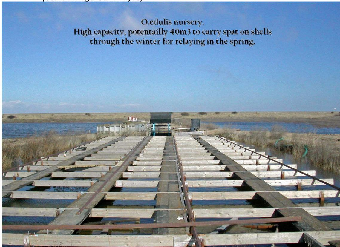
The Nursery System constructed has a 40m<sup>3</sup> capacity for rearing shellfish. The design shown is capable of rearing native oyster spat attached to cultch over the winter period for subsequent relaying the following spring.
