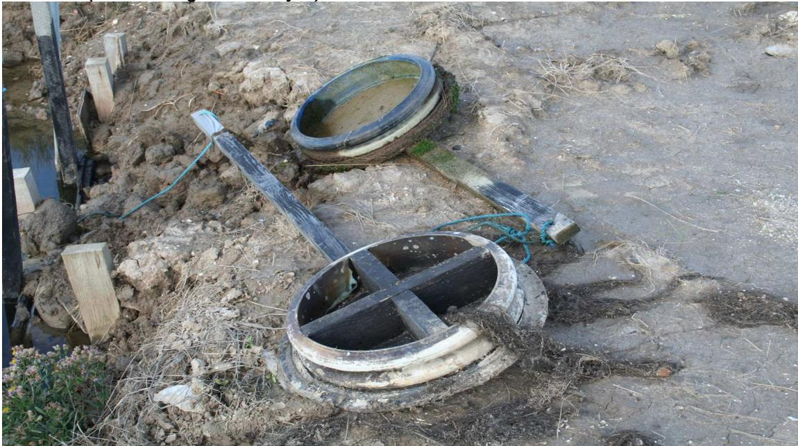
These are made from heavy duty plywood and a short section of pipe. Around the perimeter is high density black foam glued to the wood. The lower one pictured is for the female end of the pipe and the upper one, without pipe, fits the male end. The “Lollipops” have proved very practical, being lightweight and, when properly installed, completely watertight.
