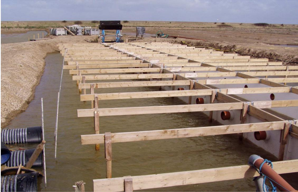
**Figure 14. Inlet and outlet system to Native Oyster Nursery System**
