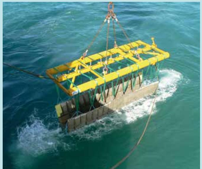
Concrete mattresses come in various forms, offering different degrees of flexibility and density to cater for different conditions and uses. But typical dimensions and weight are:
