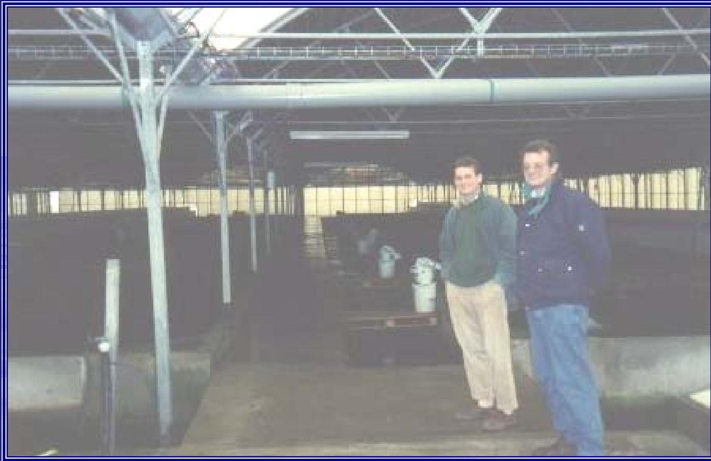
Cheaper forms of covered ongrowing units can be achieved by using “greenhouse” technology, but with rigid and opaque paneling. This unit also utilises concrete as the main construction material.
