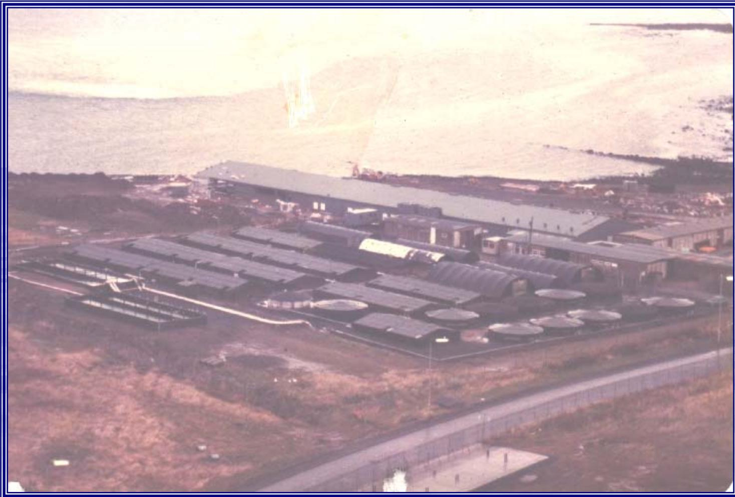
Another marine fin fish land based ongrowing unit, using a combination of circular and rectangular tanks, 0.8 m deep. All tanks have light-shading covers to prevent UV damage. Seawater is pumped on to the farm via submersible pumps at sea, coming into the header tanks on the left of the picture. It is then distributed by gravity to the main farm, via a network of PVC pipes.
